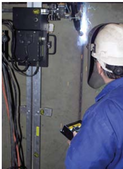
Shown Above - Vertical Weld
