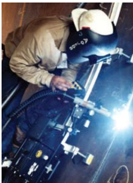
Shown Above - Vertical Weld with Linear Weaver
