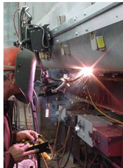
Shown Above - Overhead Weld with Pendulum Oscillator
